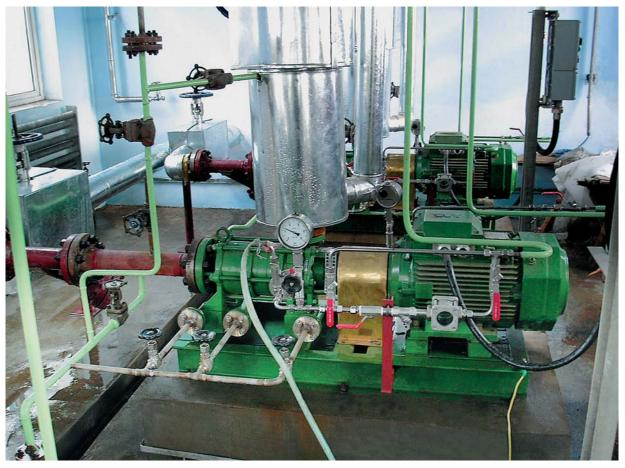
Heavy duty selfpriming Side-Channel Pumps
