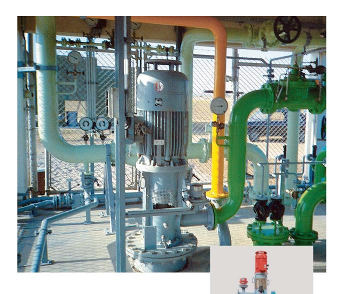
Multistage Submerged Centrifugal Pump Type HZV
