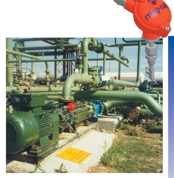
mag-safe Monitoring device for magnetic coupled pumps
