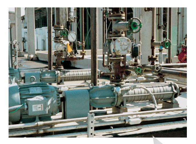
Sealless Magnetic Coupled, Heavy Duty Side-Channel Pumps our contribution for environmental protection
