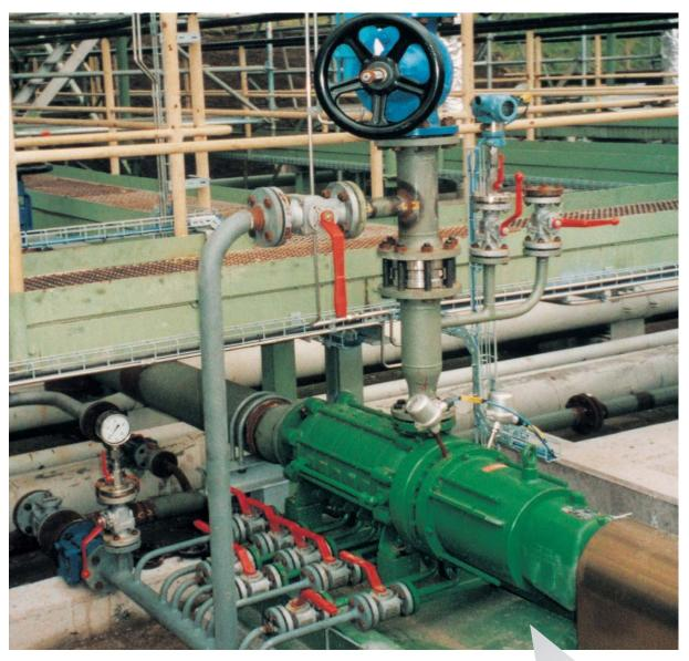
Sealless Magnetic Coupled Multistage Centrifugal Pumps Type HZM / HZMR / HZMB our contribution for environmental protection
