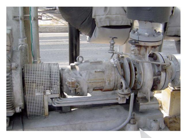
Sealless Magnetic Coupled Hot Oil Circulation Pumps acc. to DIN EN 22858/ISO 2858
